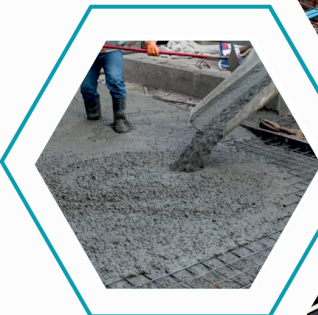
STEP 05 Concreting Process
