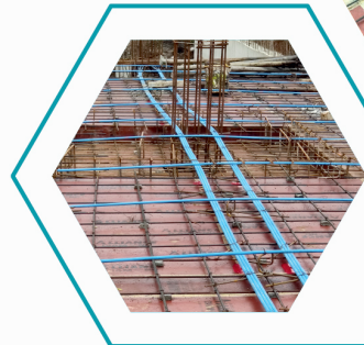
STEP 03 Installation after completion of shuttering & Bottom steel placement
